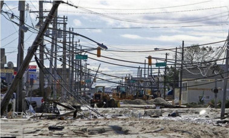
Photo: Damage from Hurricane Sandy along the Jersey Shore | Credits: nj.com
